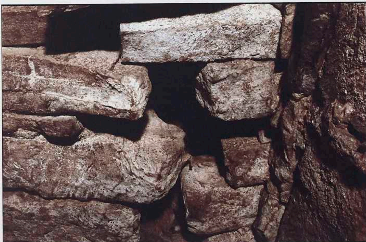
Plate 26. Collapsing arched underside of the road bridge.
