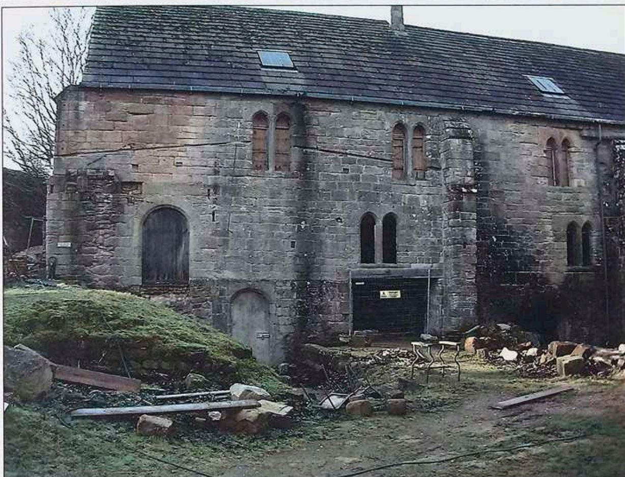
Plate 11. East wall of mill, showing roof scar.
