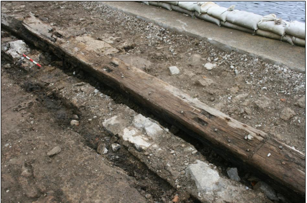
Plate 22. Lap joint foreground-right and splayed joint background-left, for upper timbers (101), around 7 metres along baseline.
