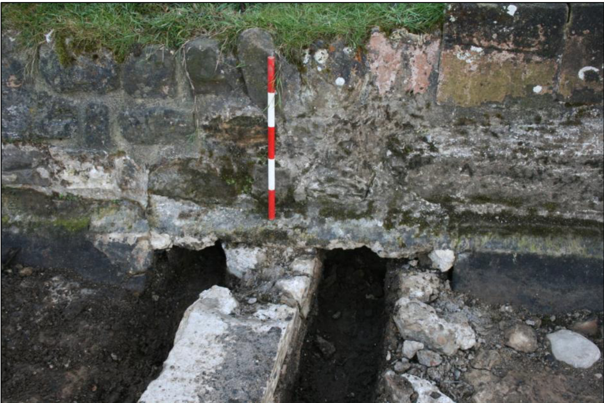
Plate 24. Channels running beneath southern dam wall, 0 metres along baseline.
