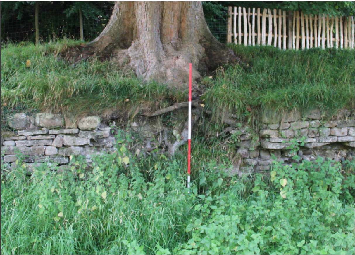
Plate 16. .South wall, detail of tree root damage.
