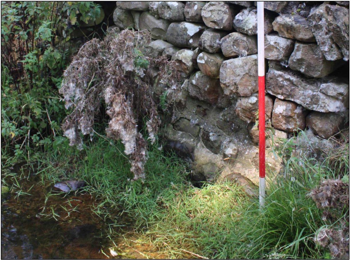
Plate 7. North wall, detail of cement render.
